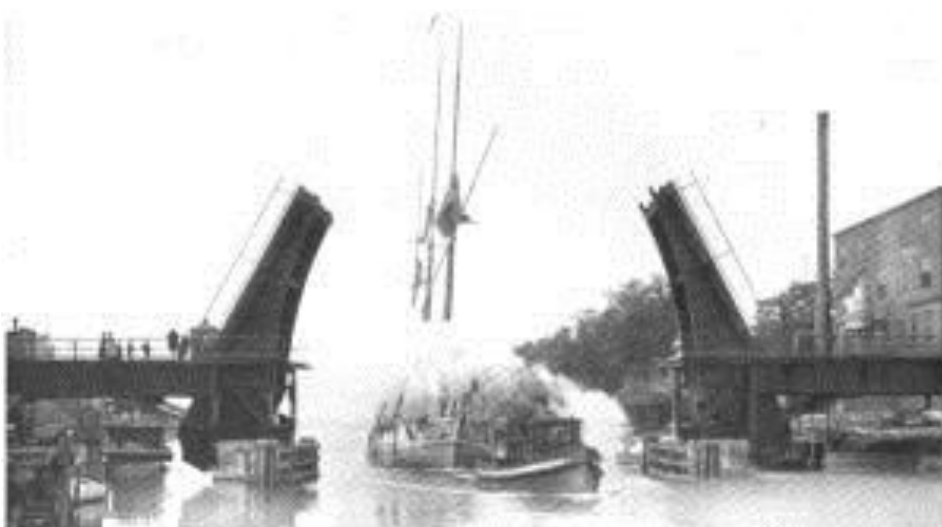
Former Maple Street Bridge, ca. 1908 Source: Scherzer Rolling Lift Bridges, 1908
